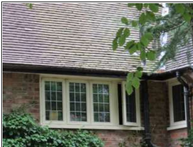
Brick Walls, Stone Slate Roof, Leaded Timber Windows
