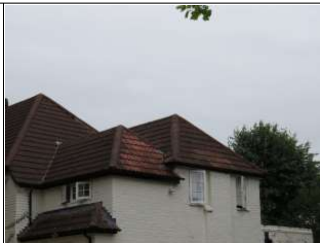
Rendered Walls and Pantile Roof
