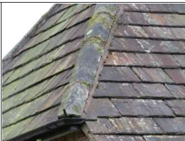
Stone Coping on Stone Slate Roof
