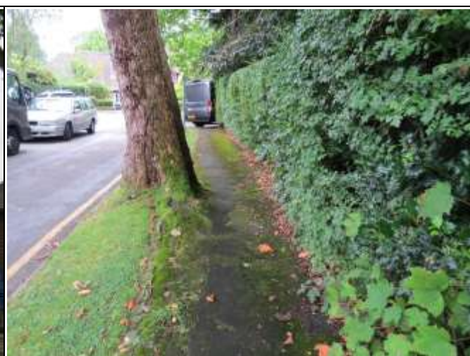
Heave from Tree Roots on Pavement
