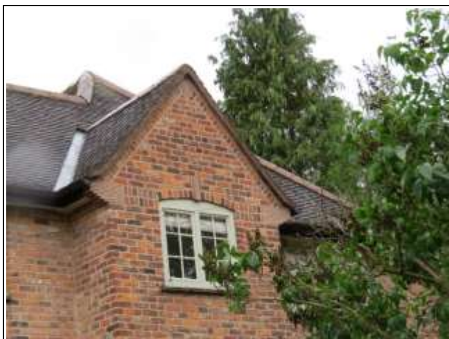
Brickwork Corbelling under Eaves and as Mosaic Effect Around Dormer
