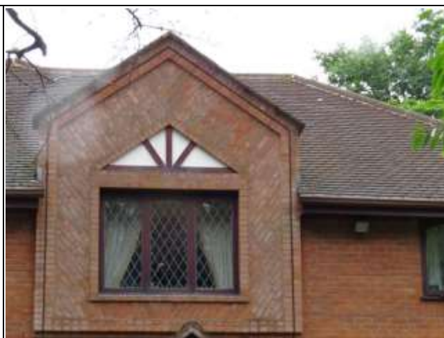
Brickwork Corbelling under Eaves and as Mosaic Effect Around Dormer
